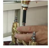
Step 2: Use 13mm Wrench to remove the pull-down tube
