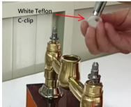
**Step 3:** Remove the defective tube and put in a new tube inside the spout
