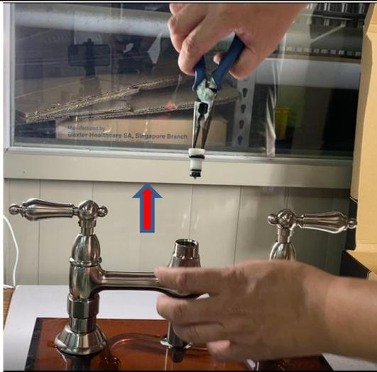
Using needle nose plier pull diverter out.
